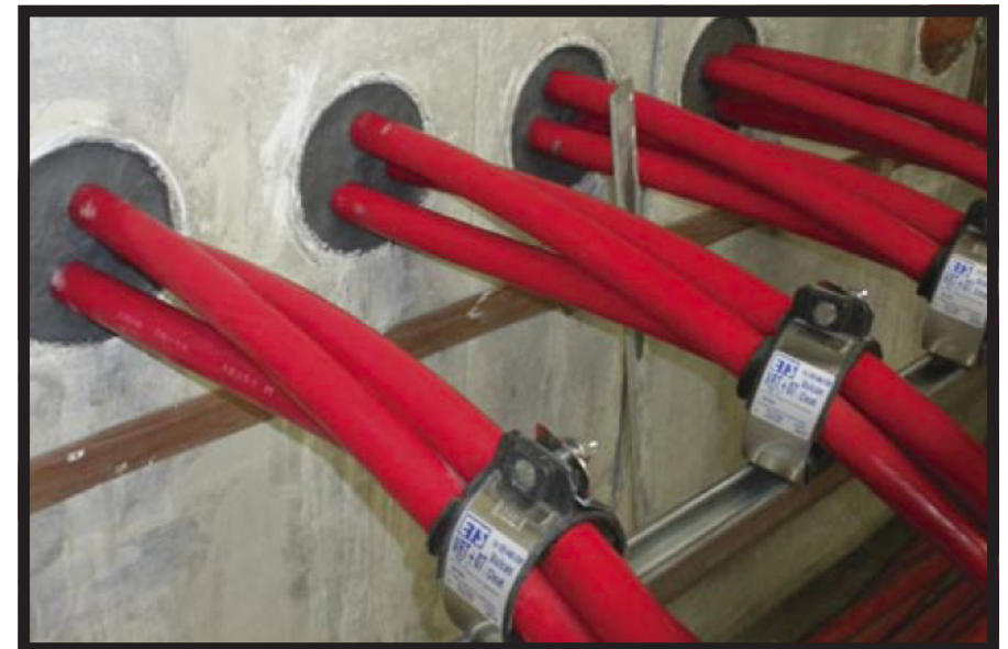
Cable duct seal © Aquobex
