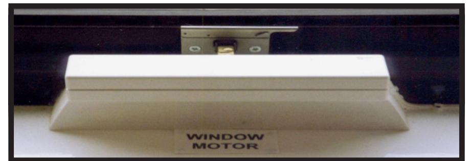
Automated opening system for water inlet (2) © BRE
