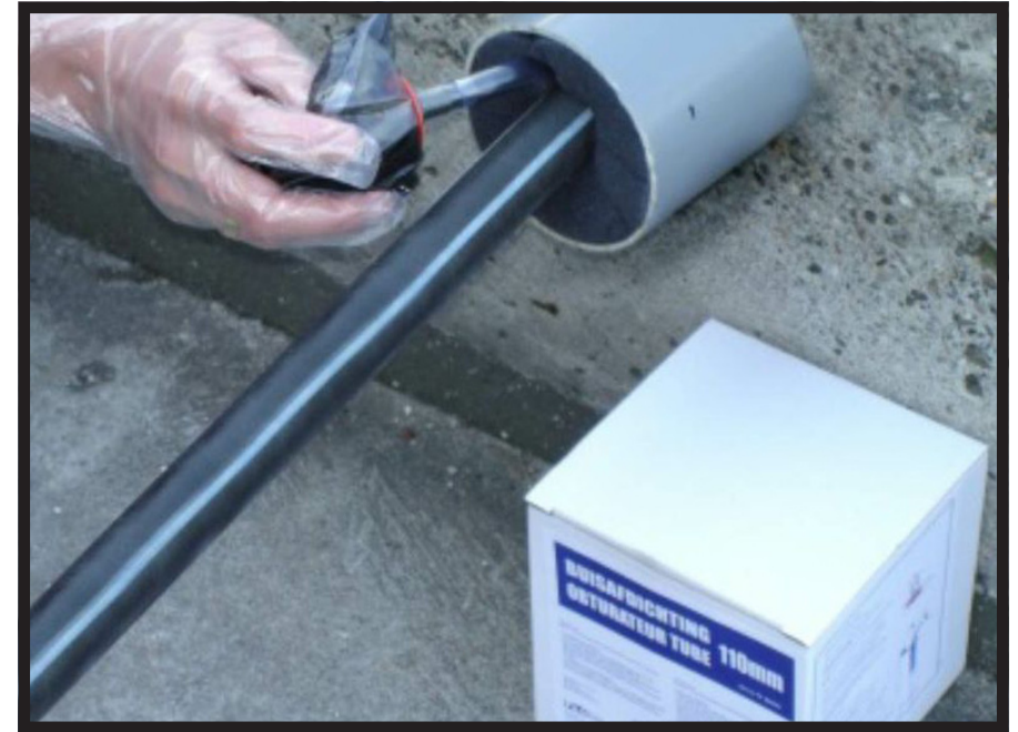
Duct sealing system © Aquobex
