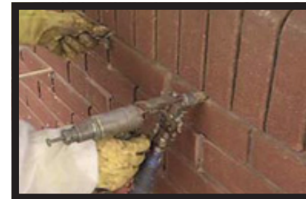
Closed cell polyurethane cavity wall insulation, injection process (2)
