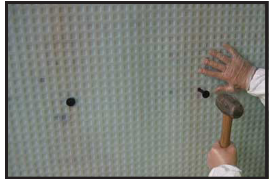
Cavity damp proof membrane (1) © Triton Systems
