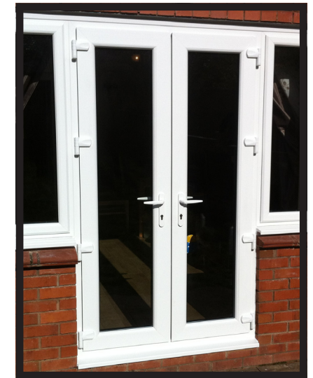
Flood resistant PVC-U french door © Aquobex
