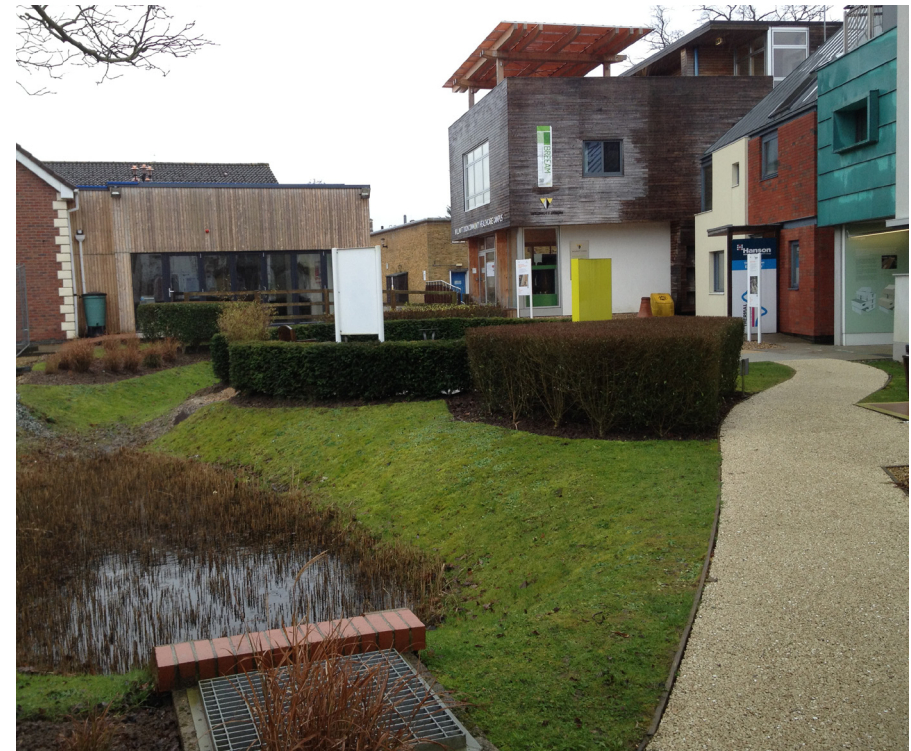
BRE Innovation Park © BACA Architects
